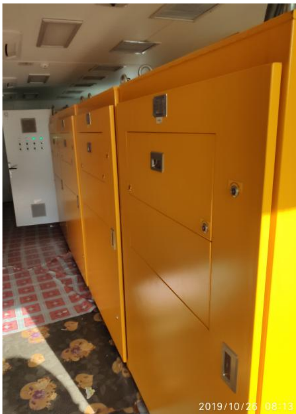
Vibroflot Inverter Control Cabinet in Cabin
