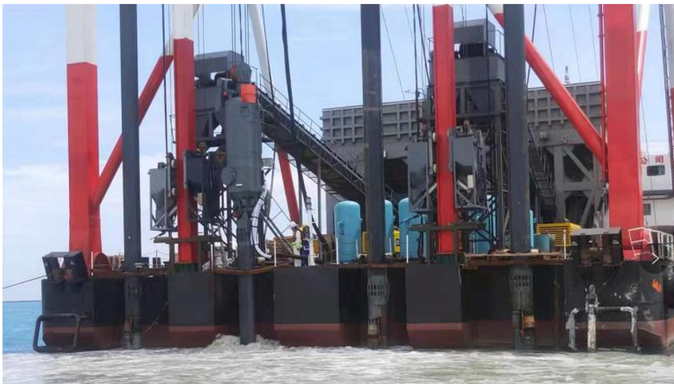
BF vibroflots in underwater boring
