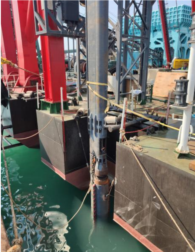
BF Vibroflots Dipped into Sea Water
