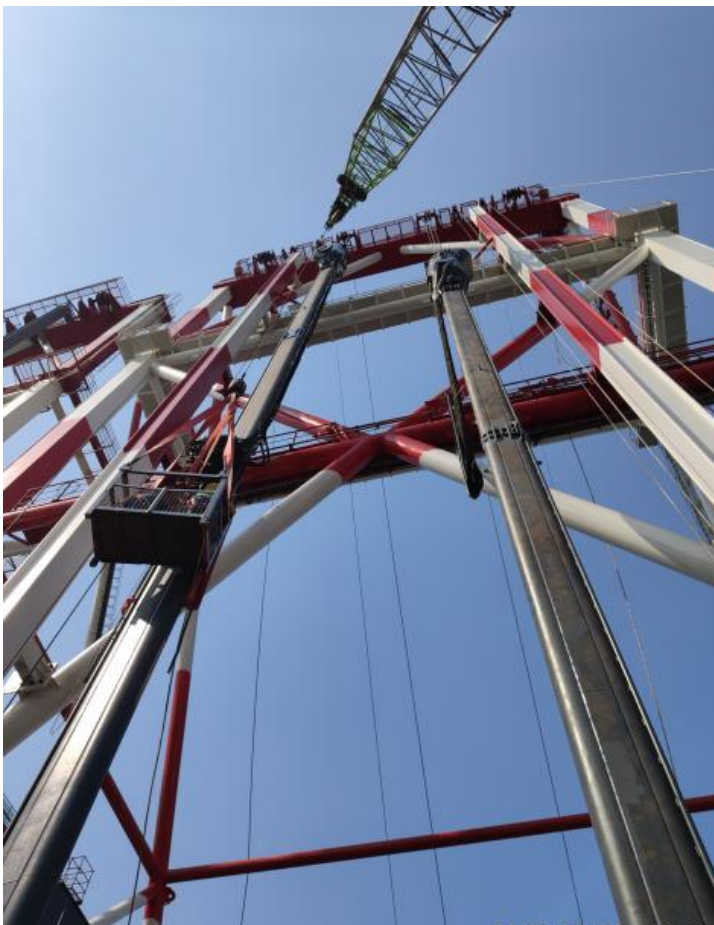
BF Vibroflot in assembly and installation
