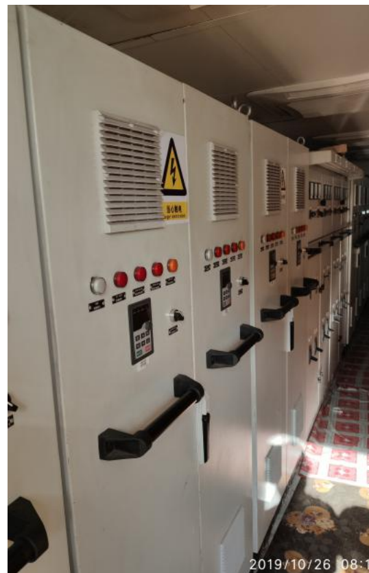
Construction Quality Management Control Cabinet in Cabin
