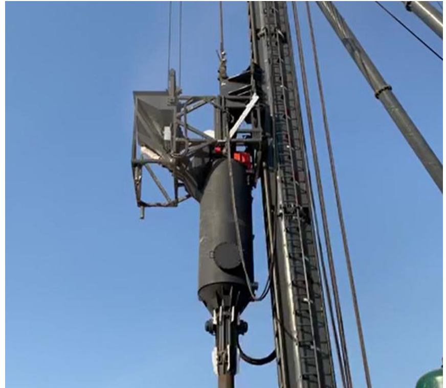
Feed stone to container and start to make pile
