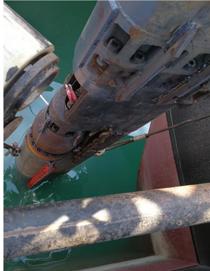
BF Vibroflots Dipped into Sea Water
